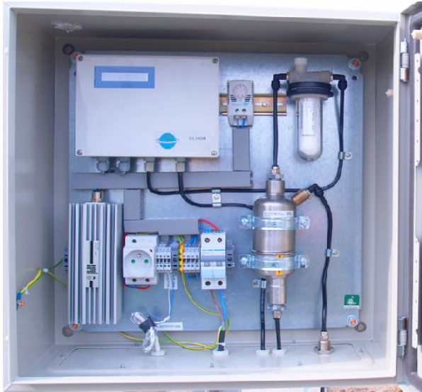
Ambiant H 2 S analysis Based on Small IRM750 analyser Small cabinet with gas sampling
